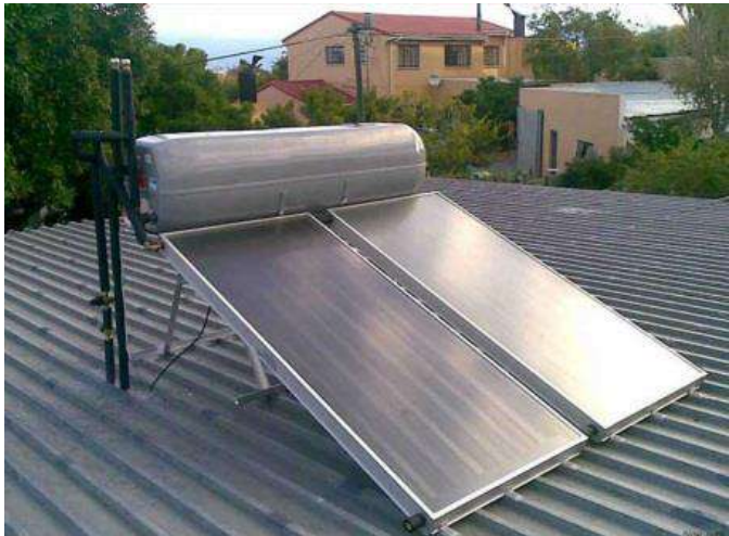
Gambar 2.4 Model umum roof solar water heater [22]
