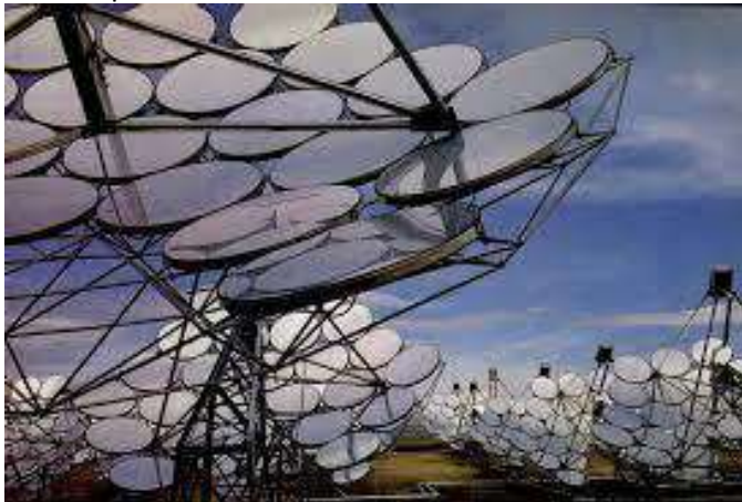
Gambar 6.9 Plant La Jet solar dish system di California dengan 700 unit dish [60]
